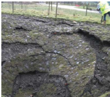
Shaft collapse
