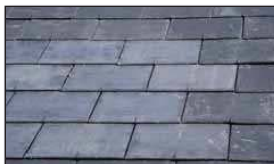
PV Roof Cladding replicating the appearance of slate
