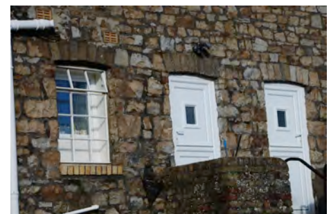
Traditional steel window which is appropriate adjacent to new white uPVC doors that are not. Note also inappropriate white uPVC pipework.
