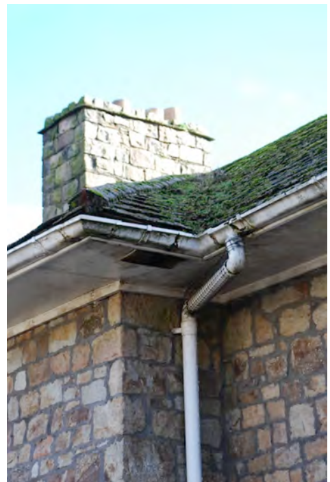
Detail of existing roof / eaves arrangement. The existing tiles attract excessive moss growth. The plain soffit and large diameter downpipes are inappropriate details in the context of Bute Town's heritage.
