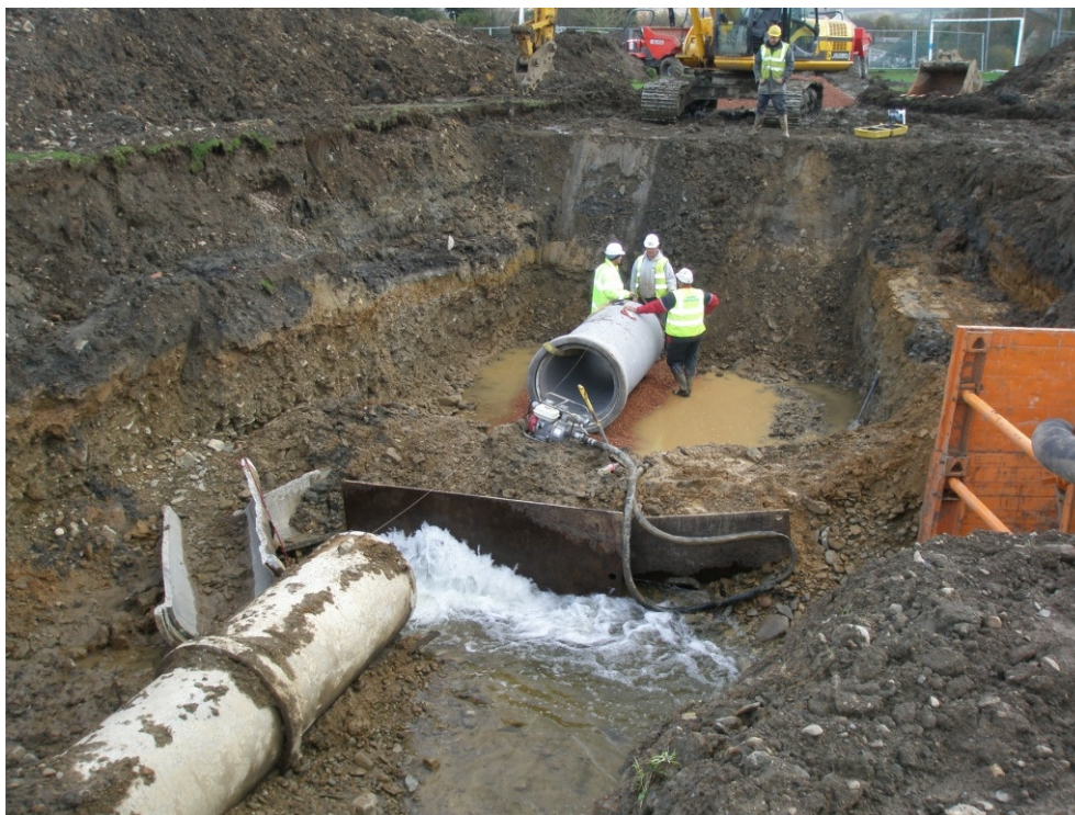
Sub-standard culvert being replaced
