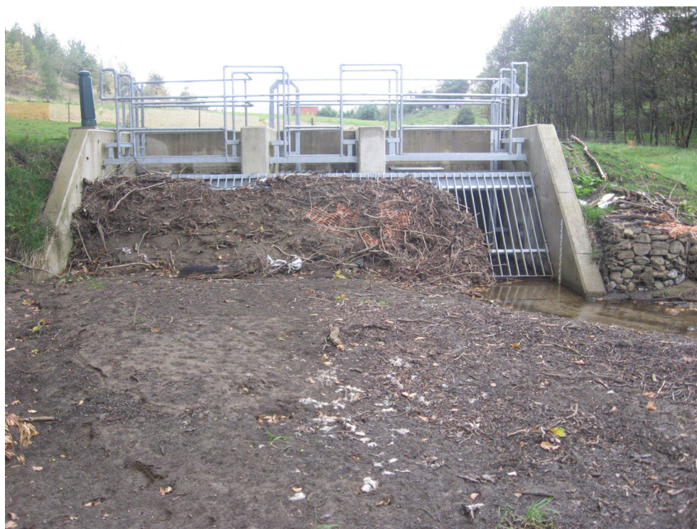
Blocked grid following heavy rain
