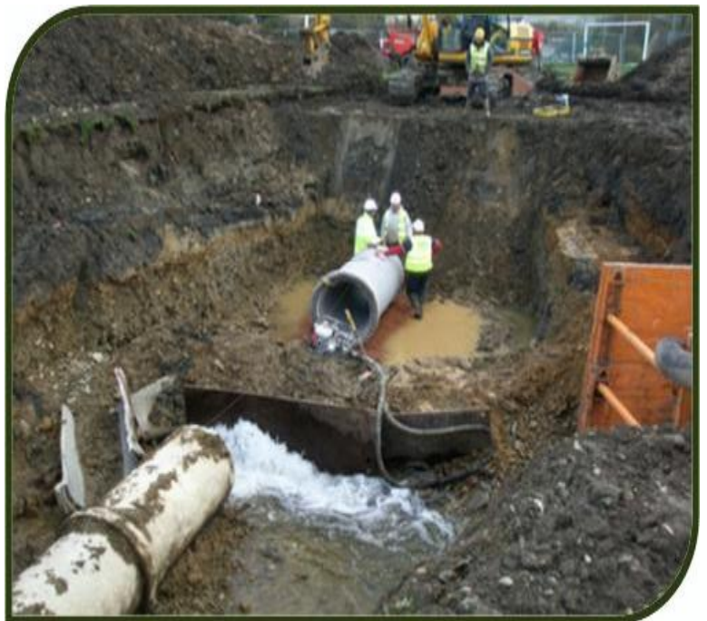
SUB-STANDARD CULVERT BEING REPLACED
