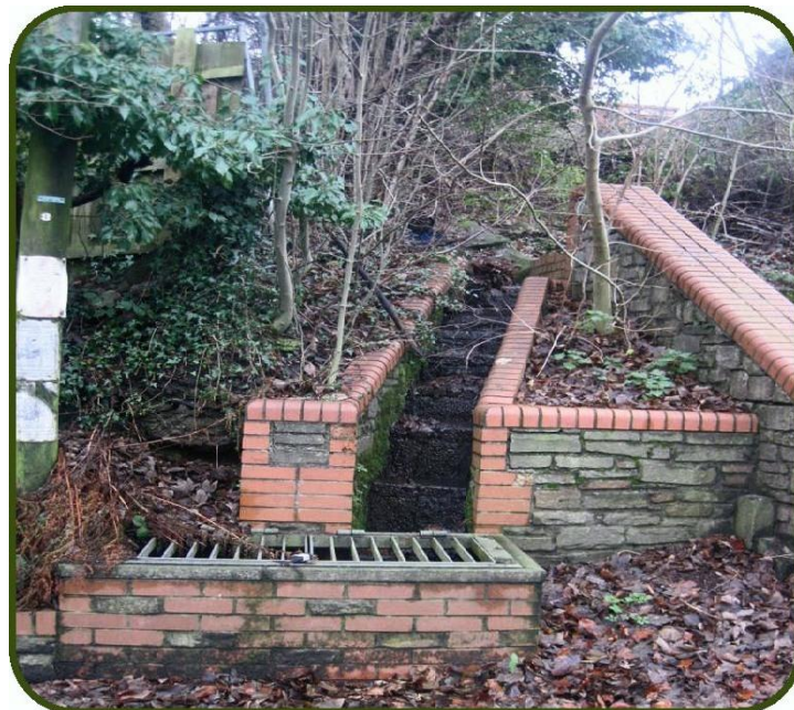
CASCADE AND INTAKE STRUCTURE IN CRUMLIN
