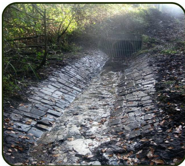
STONE PITCHING DRAINAGE CHANNEL AT BARGOED
