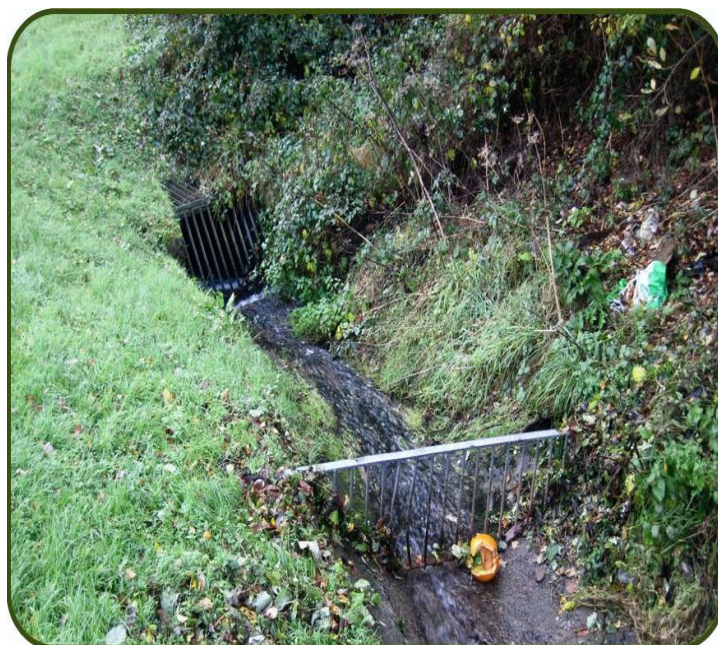
SECONDARY TRASH SCREEN AND CULVERT INTAKE STRUCTURE AT BLACKWOOD
