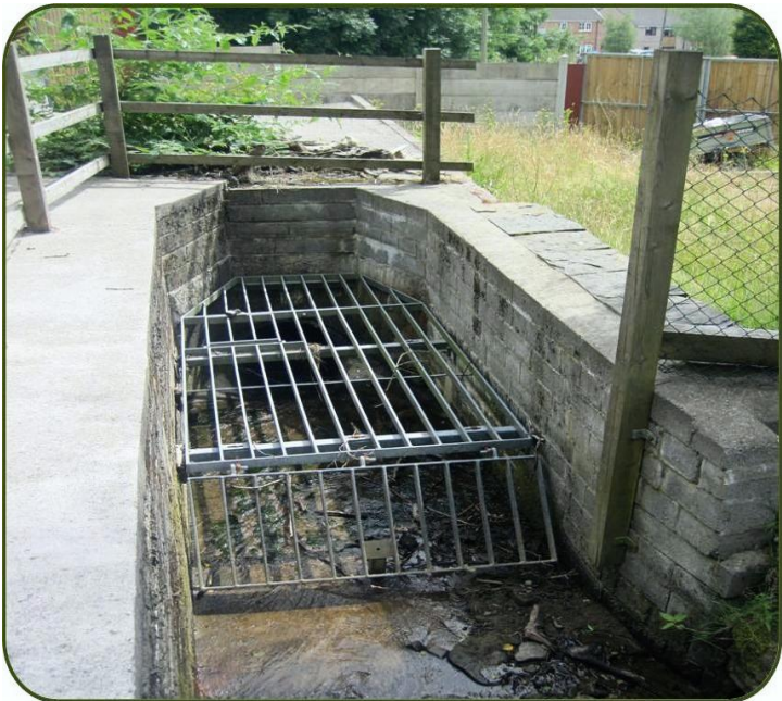
INTAKE STRUCTURE IN ABERTRIDWR
