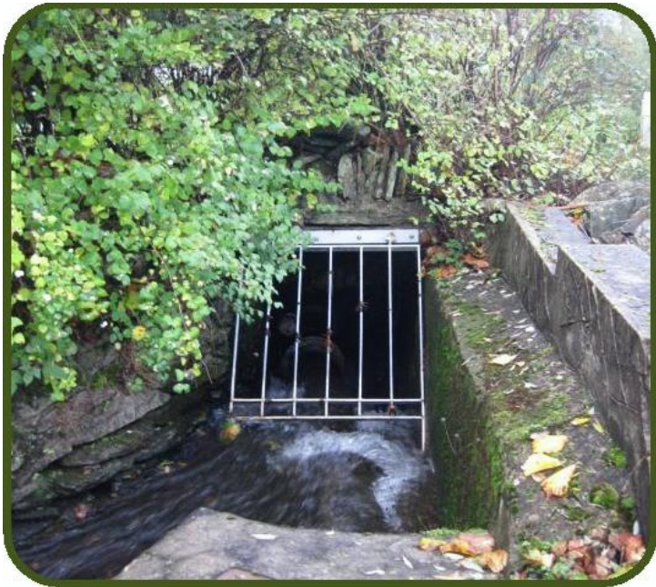
HEADWALL STRUCTURE IN PENGAM
