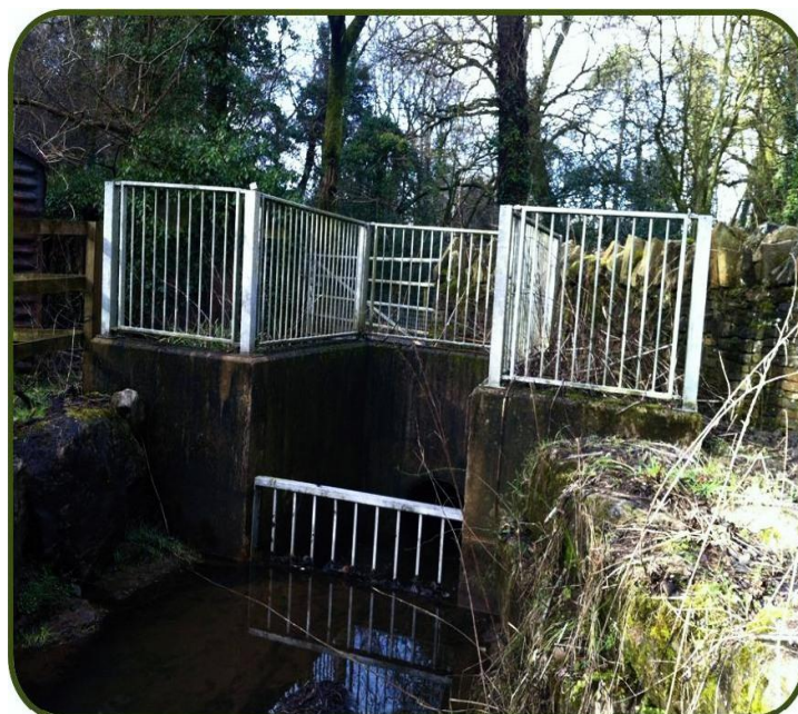
SECONDARY TRASH SCREEN AND HEAD WALL IN CAERPHILLY SOUTH
