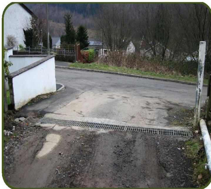
HEAVY DUTY DRAINAGE CHANNEL TO CAPTURE SURFACE WATER RUN OFF IN MARKHAM
