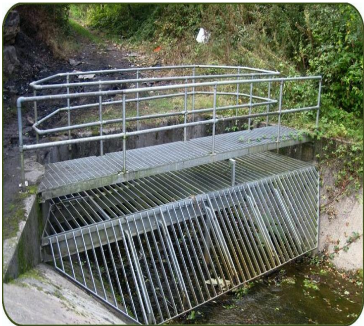
CULVERT HEADWALL AND TRASH SCREEN IN NEW TREDEGAR
