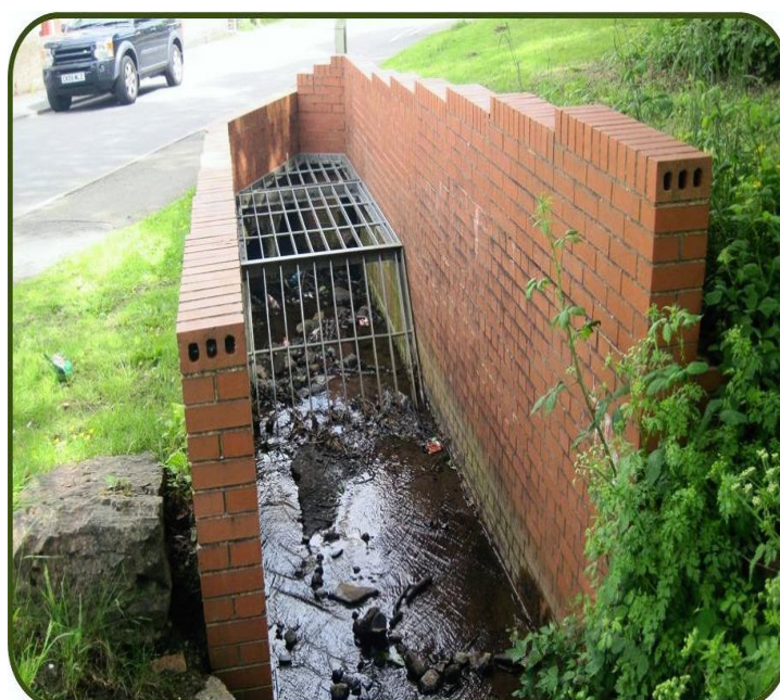
INTAKE STRUCTURE IN MAESYCWMMER
