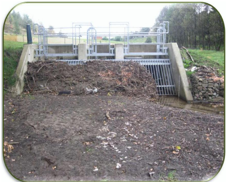
Blocked Grid Following Heavy Rain
