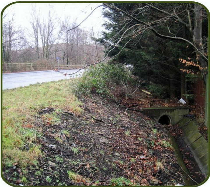
LINED CONCRETE DITCH LEADING TO CULVERT AT CAERPHILLY EAST
