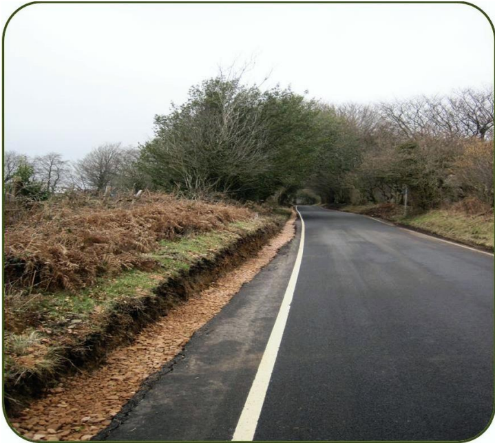
FILTER DRAIN TO THE EDGE OF THE CARRIAGEWAY IN MANMEOL
